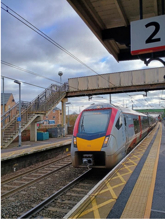
The old footbridge at Stowmarket
