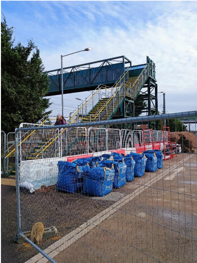
The worksite compound
