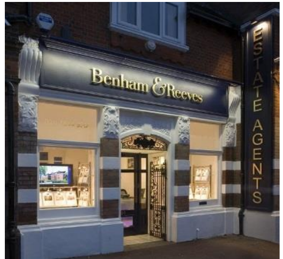
Cornice incorporating recessed lighting
