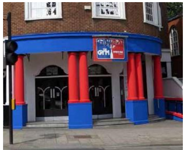
Inappropriate use of visually dominant colours
