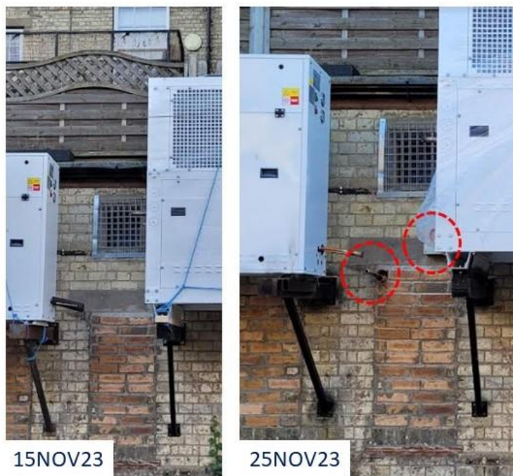
Figure 1: Electrical switch and pipes installation through the walled windows.
