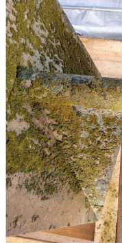
deep gaps found around bell housing and stonework/loose flints
