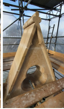
deep gaps found around bell housing and stonework/loose flints
