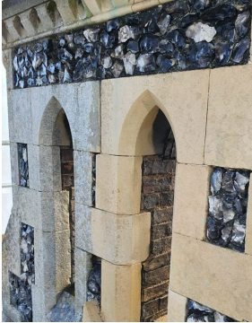
before and after cleaning and repointing
