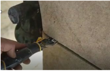
deep gaps found around bell housing and stonework/loose flints
