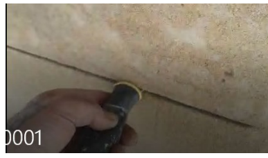
deep gaps found around bell housing and stonework/loose flints
